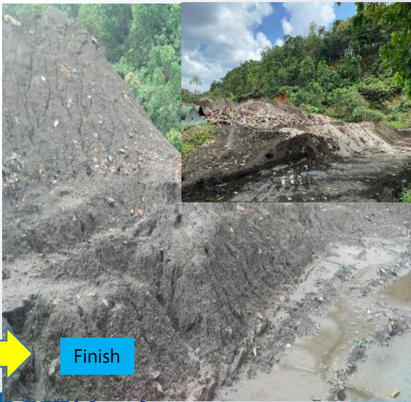
1 Leveling of the solid waste cover layer
